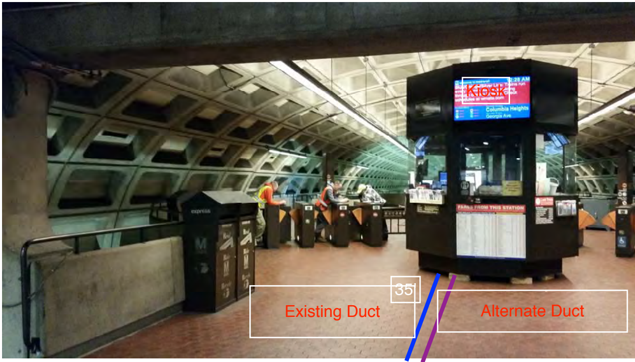
Photo 1 – Existing and alternate duct layout on mezzanine floor
